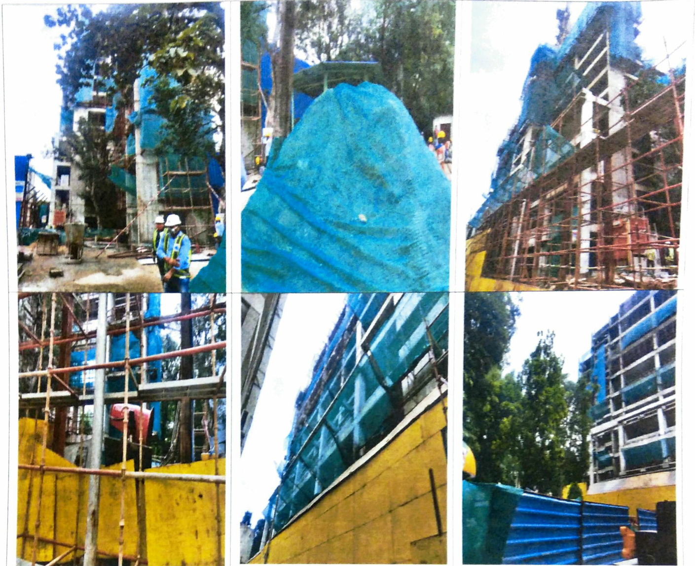
Photos 1 to 6: Ongoing Construction Work, Scaffolding, Anti Smog gun, etc.
